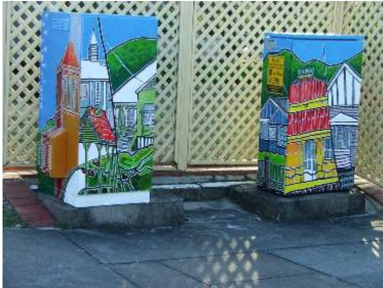
Painted Energex Boxes Ashgrove
